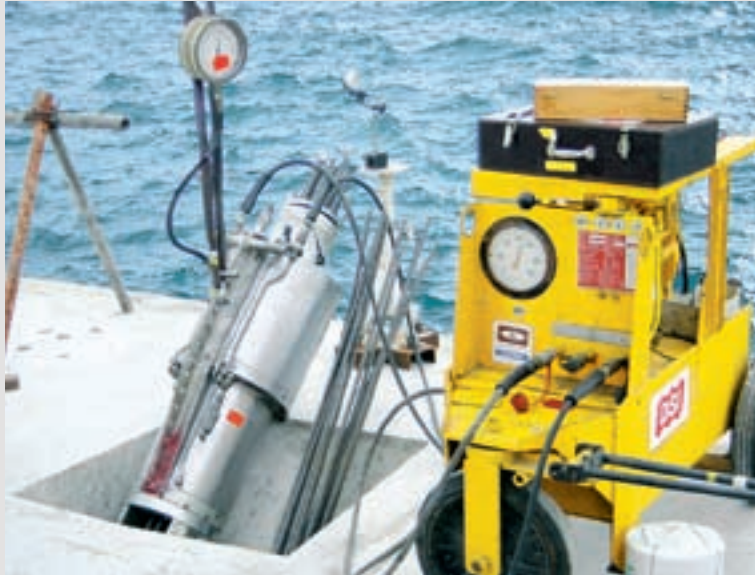
Tensioning of the DYWIDAG Multistrand Anchors
