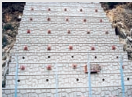
Top and right: Stabilized slopes with DYWIDAG Threadbar Anchors
