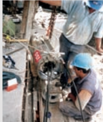
Prestressing tests performed on the anchors
