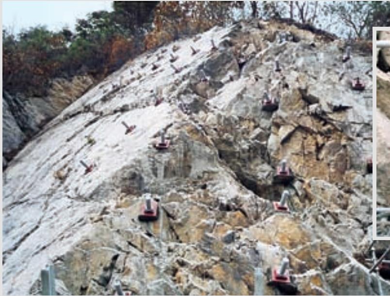
Slopes secured with DYWIDAG Threadbar Anchors
