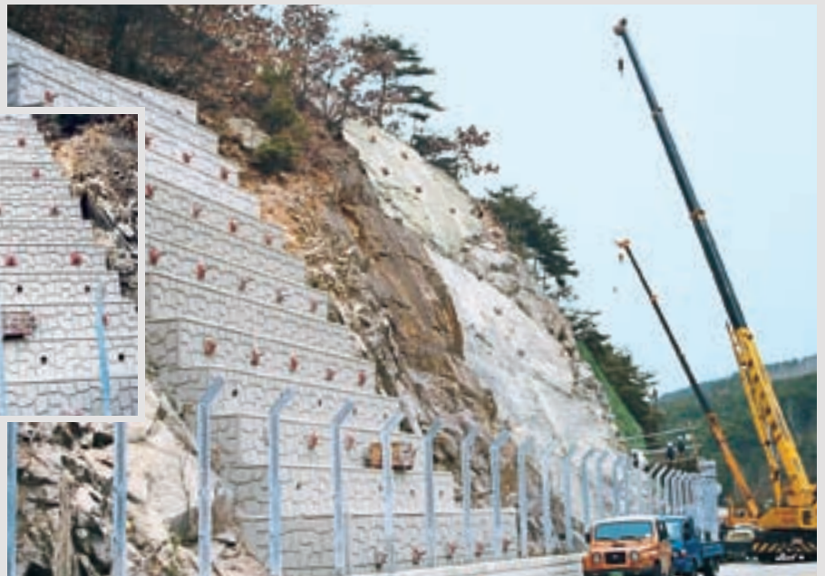
Top and right: Stabilized slopes with DYWIDAG Threadbar Anchors
