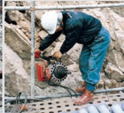
Stressing of the anchor with DYWIDAG Jack
