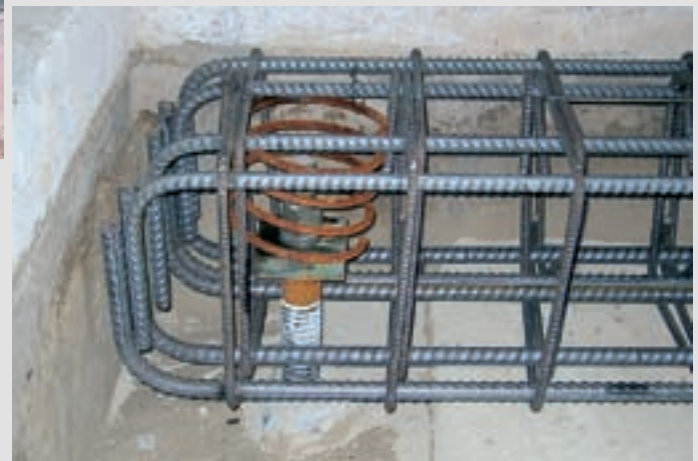
Detail view of GEWI® Pile head (compression)
