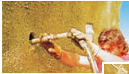
Grouting through hollow core
