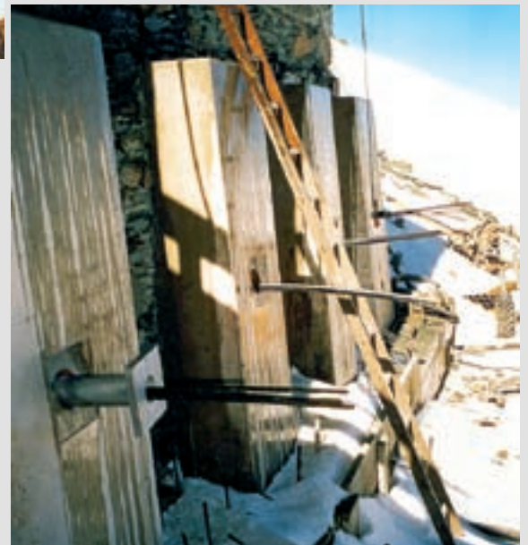
DYWIDAG Strand Anchor after installation
