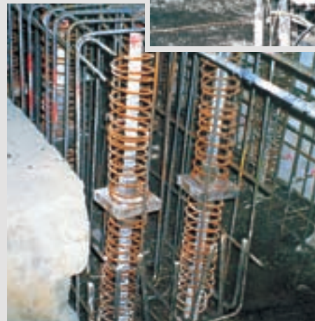
Detail view of GEWI® Pile head (compression/tension)
