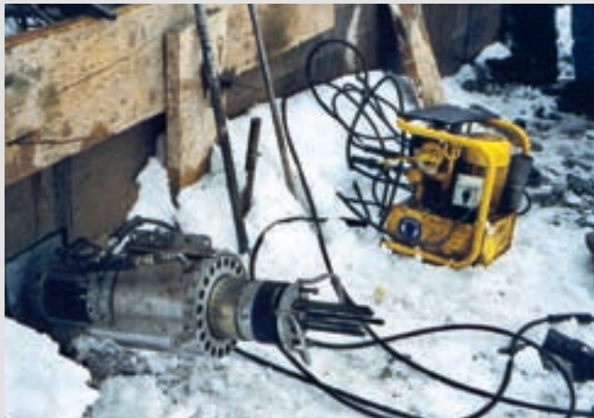
Tensioning of the DYWIDAG Strand Anchors
